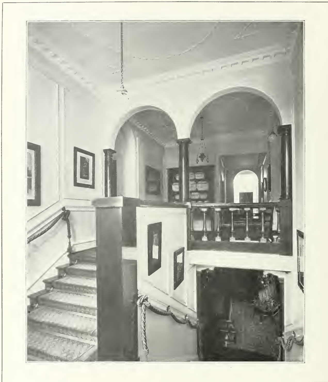
The woodwork is mahogany, and the walls are panelled in Parian cement.
